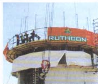
Silo 1 at Impala Platinum's no. 20 shaft in progress.
