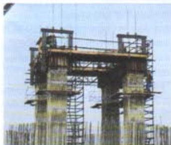
Slip form construction of columns.
