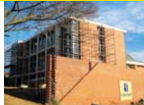
The upgrade of and extensions to the Chatsworth police station
