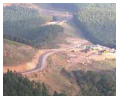
Construction of new road in the Barberton area
