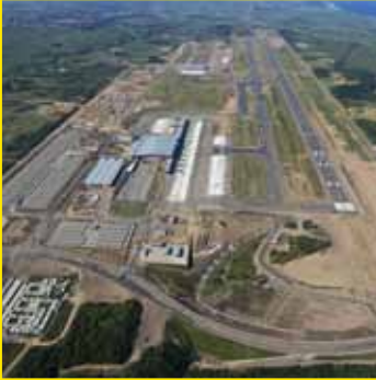
Civils work at the new King Shaka International Airport
