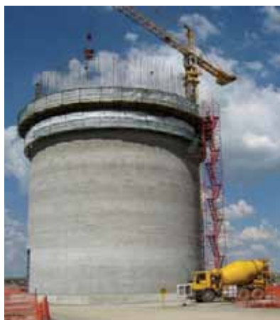
Construction of an 18 meter diameter, 50 meter high silo in Balfour, Mpumalanga
