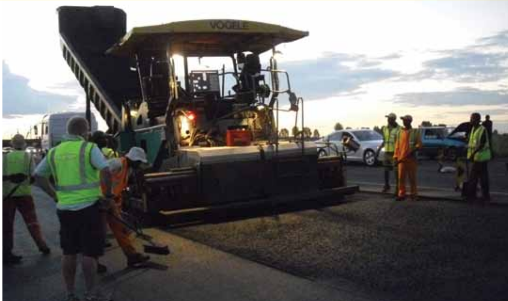
Surfacing of N8 near Bloemfontein Airport.
