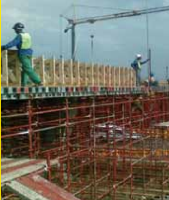
N8 road – 82 meter long double dualway concrete bridge
