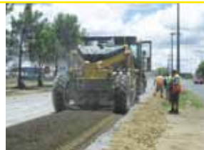
N8 interchange at the Bloemfontein Airport
